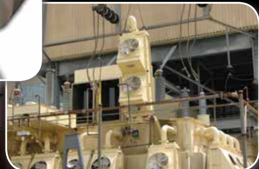
Installation of a T-REX
